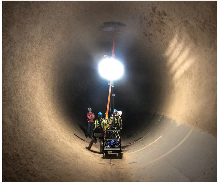
An assessment crew inside the 21-foot diameter Salt River Siphon.
