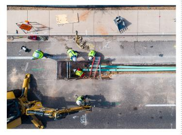
Our Beardsley WRF Solids Pipeline Rehabilitation project for the City of Peoria has been selected as the AZ Water Association's 2020 Wastewater System Project of the Year. This project involved the installation of the longest section of sliplined fusible PVC pipe ever completed in Arizona. Visit our website for more project information and photos.
