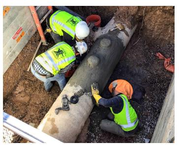
Achen-Gardner completed an emergency repair on an 18" welded steel transmission main on Gilbert Road as part of our **Wet Utility Emergency Repair Services JOC for the City of Mesa**. **See our website for more project details and photos**.
