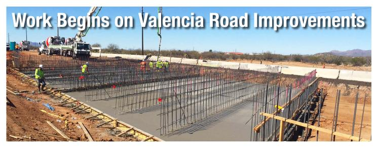
Achen-Gardner crews constructing one of six box culverts as a part of our Valencia Road (Mark Road to Wade Road) Design-Bid-Build project in Pima County. The new box culverts will improve drainage along the corridor.
